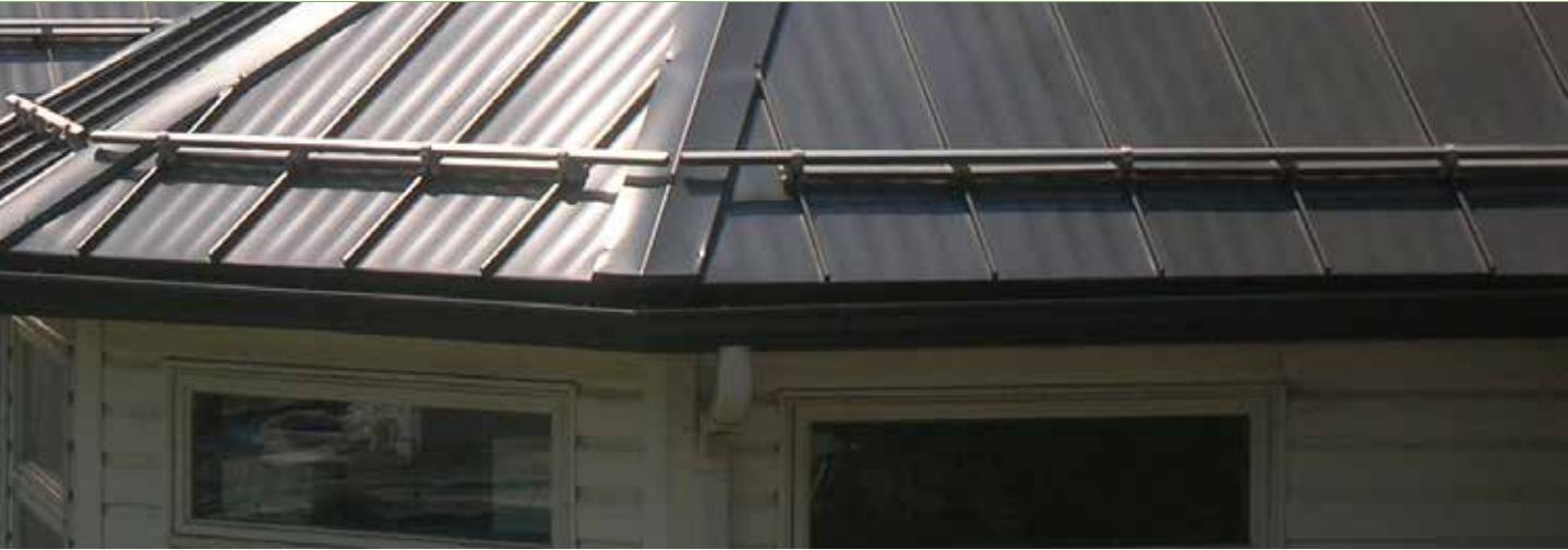
This roof features Antique Bronze with Snow Retention System.
