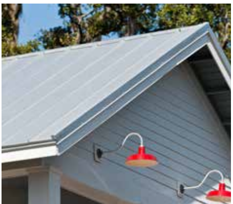
1 1/2" SSR in Acrylic Coated Galvalume, selected for its reflective qualities, covers the roof of this home.
