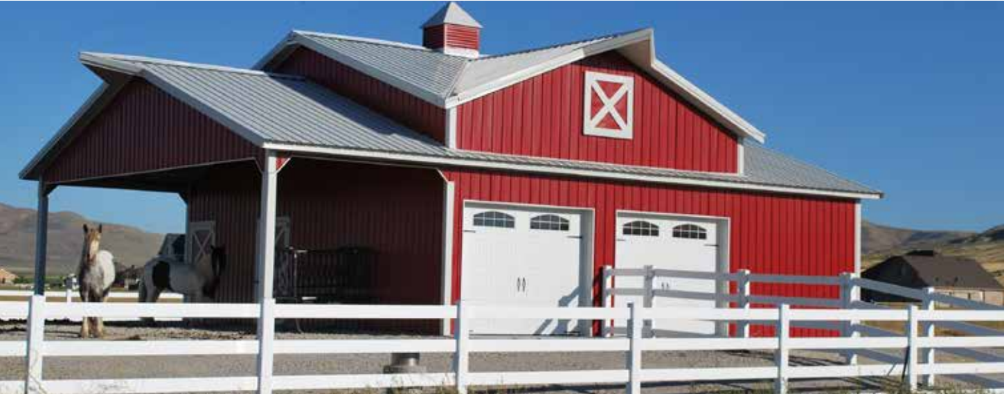
Grandrib 3 Plus covers the roof and walls of this barn.
